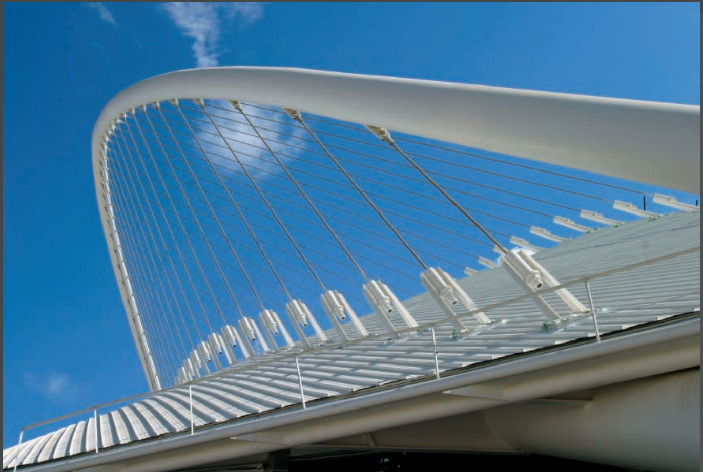
• ATHENS, GREECE -- VELODROME pot bearings for the roof covering
