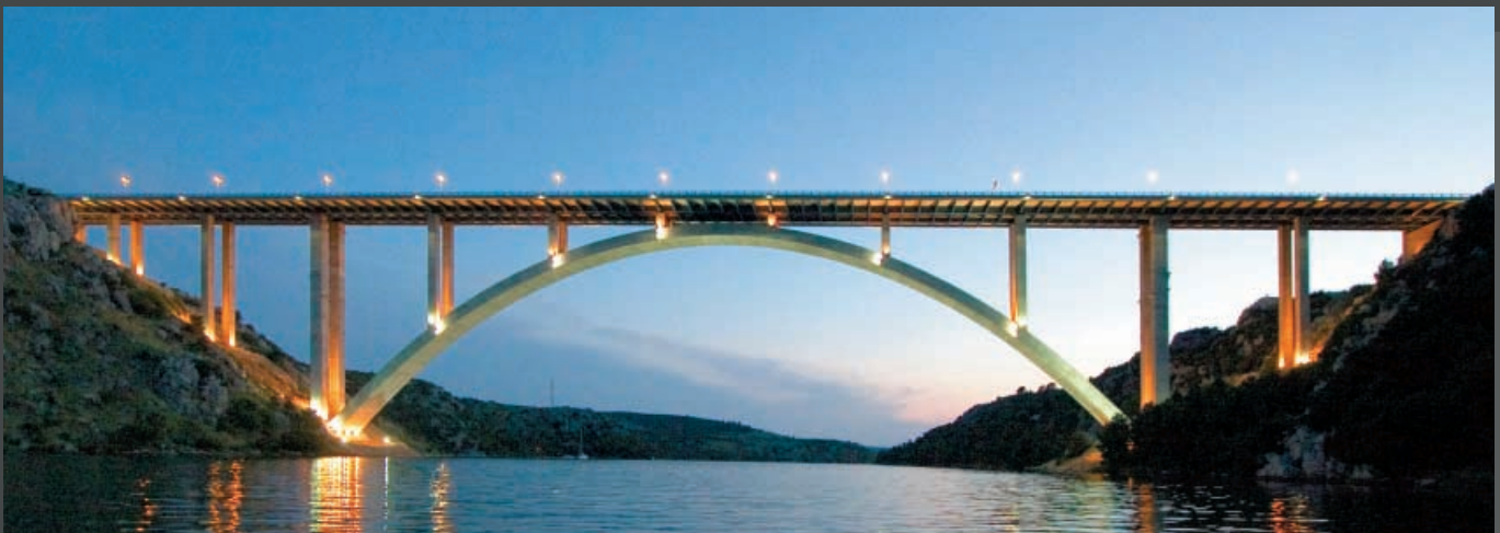
• CROATIA -- KRKA BRIDGE pot bearings with fuse restraints
