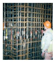
Rotate the locknut along the continuation bar to abut the coupler.
