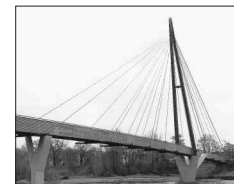
Bridge over Cracauer Wehr, Pylon Stays
