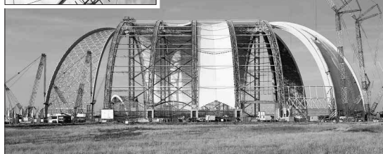
Cargo-Lifter, Brand, Transverse Bracing
