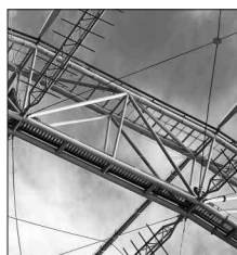
Cargo-Lifter, Brand, Transverse Bracing
