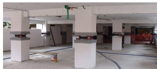
Retrofitting of PS isolators
