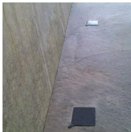
Void formers shown at Slab-to-Wall joint
