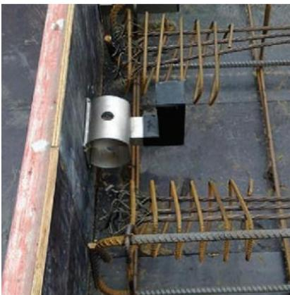
HLDQ-L30 Sleeve nailed to formwork
