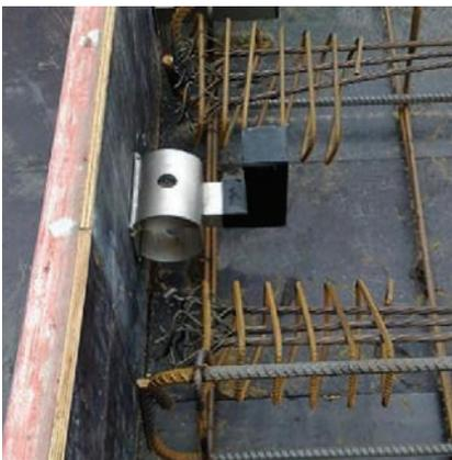
HLDQ-L30 Sleeve nailed to formwork
