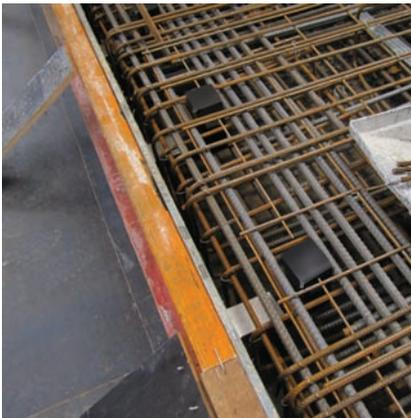
Reinforcement being located around ESDQ-L20 Sleeves
