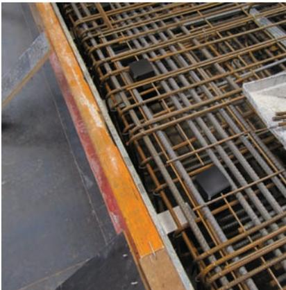
Reinforcement being located around ESDQ-L20 Sleeves
