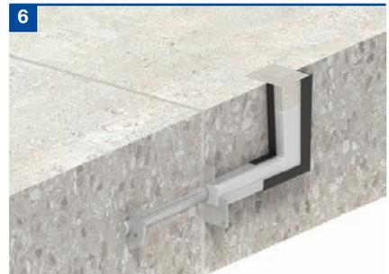
After 24 hours the void former can be filled with cementitious material, level with the top of the slab, to complete the installation.
