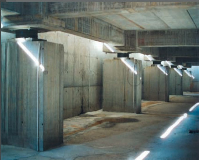
UDINE, ITALY - "Gervasutta" Hospital: installation
