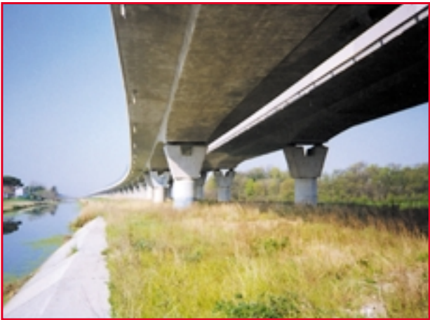
Coltano Viaduct - Italy
