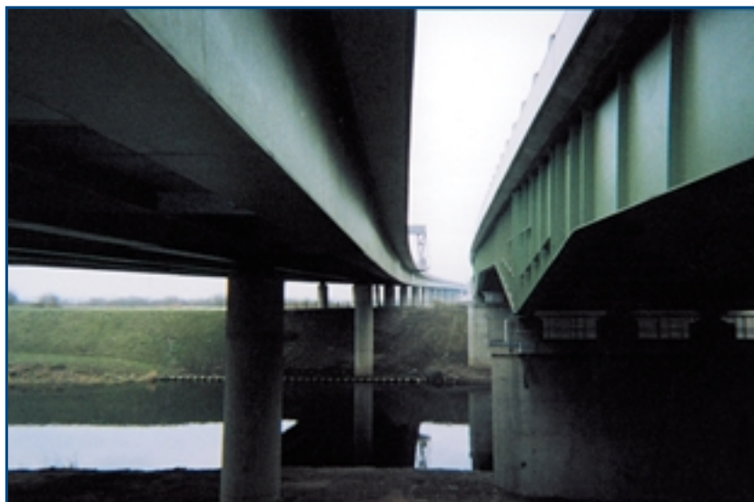
New Thelwall Viaduct - UK
