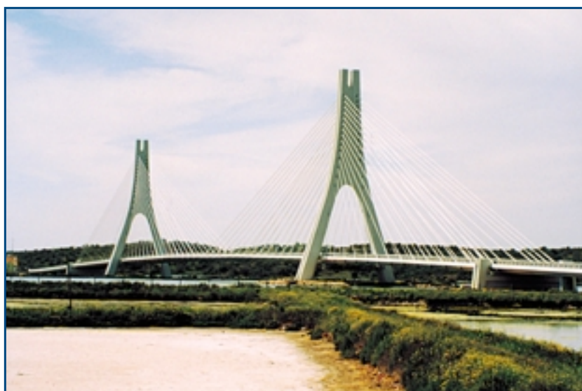
Portimao Bridge - Portugal
