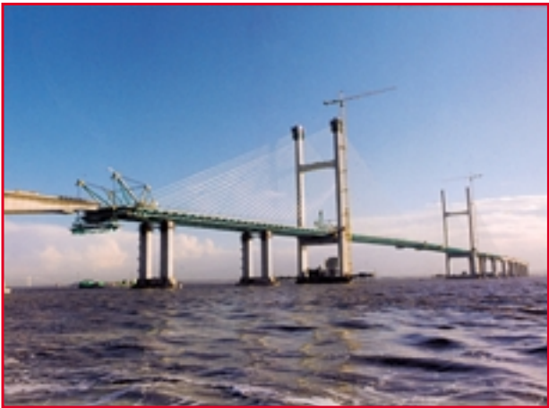
2nd Severn Crossing - UK
