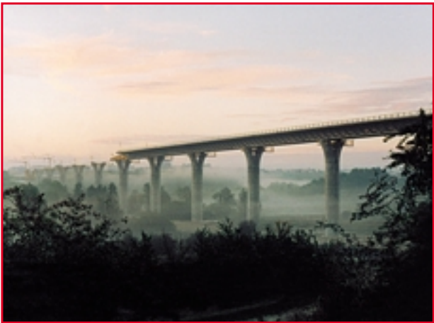
Scardon Viaduct - France
