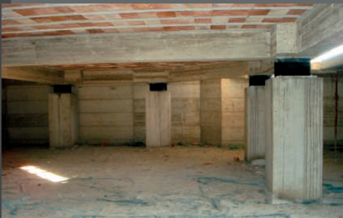
• ANCONA, ITALY - "La Torre" office building: installation
