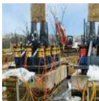
Vorspannen eines Seiles mittels Hydraulik-Spannvorrichtung Pretensioning of a cable with hydraulic tensioning system
