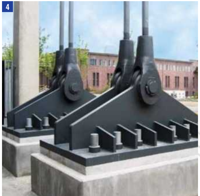
Anschluss Abspannseil am Fundament Connection of stay cable to foundation
